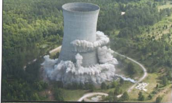
An aerial view of the K Cooling Tower demolition.
